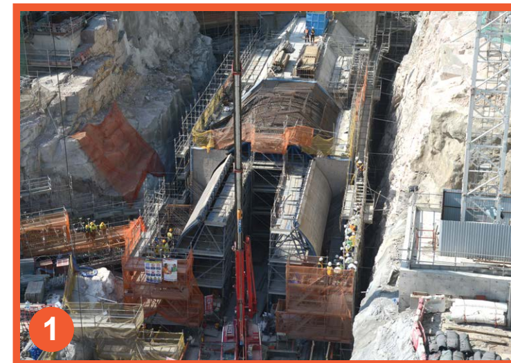
以明挖回填法興建的隧道 Underpass constructed by cut-and-cover method
